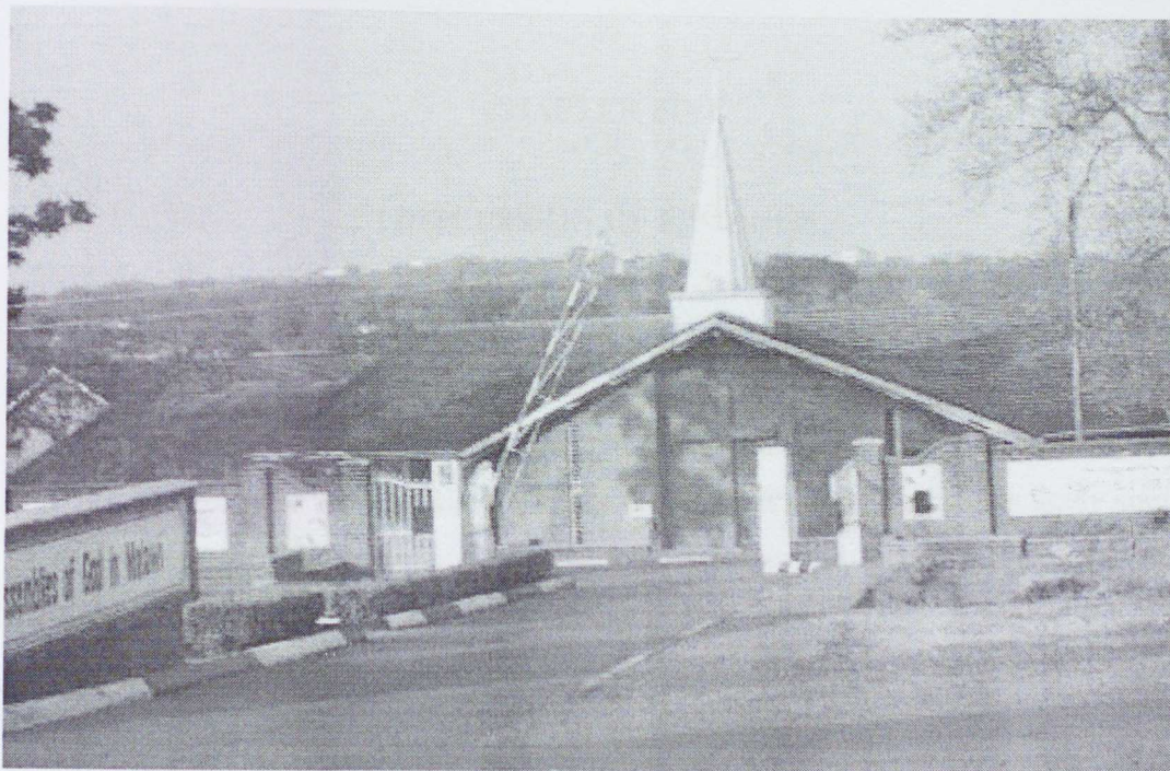
Figure 6: Malawi Assemblies of God Sheaffer Complex, Housing the National Headquarters, the MAGIT and the MAGU
